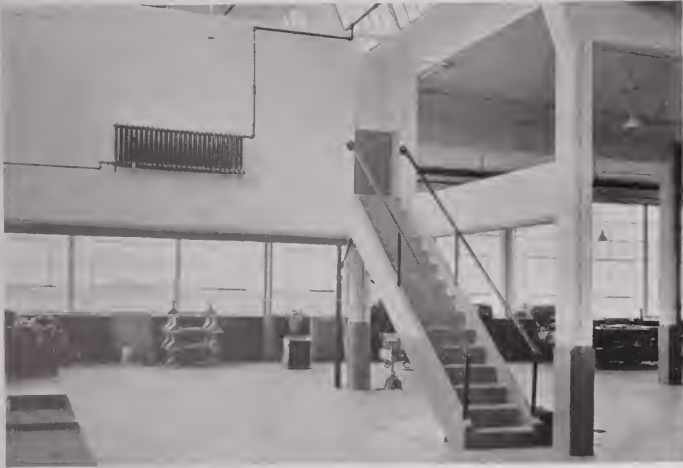
TOILETS LOCATED ON BALCONIES Conveniently Accessible But "Out of the Way"
